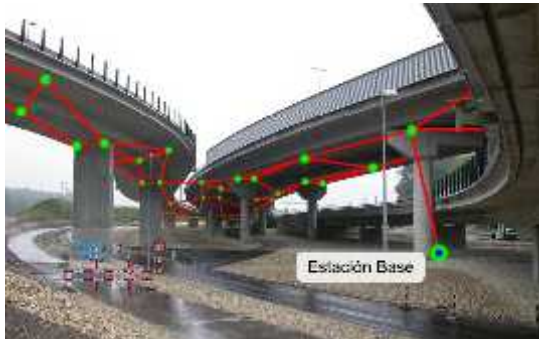
Figure 2: QDSN application example, bridge monitoring.
